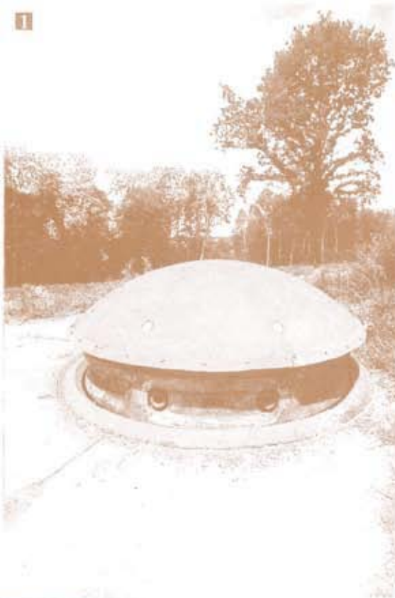
1. Turret of 75 with eclipse infortified position 2. Entrance and ditch : In the foreground, the bridge In the middle distance one caponnière 3. Western yard, with the reinforcement in special concrete made in 1884. 4. Blockhouse of Easter (model Bourges).
