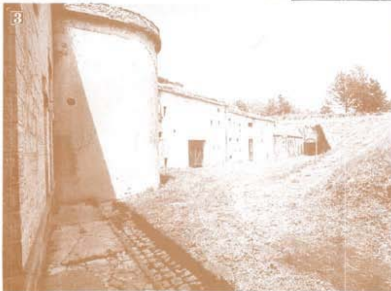
1. Turret of 75 with eclipse infortified position 2. Entrance and ditch : In the foreground, the bridge In the middle distance one caponnière 3. Western yard, with the reinforcement in special concrete made in 1884. 4. Blockhouse of Easter (model Bourges).
